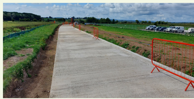
Improved quality of the flattened concrete finish
