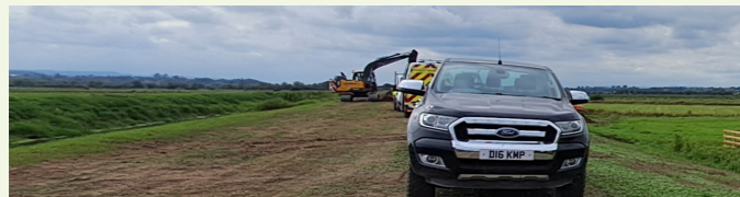
Work at the River Tone embankment
