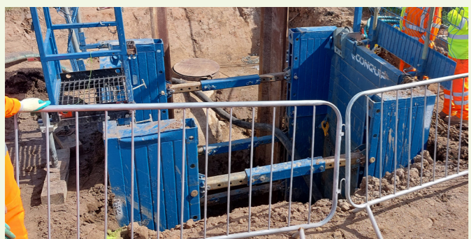
Installation of trench boxes
