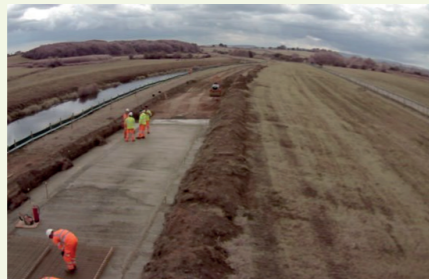
Construction of Hook bridge spillway
