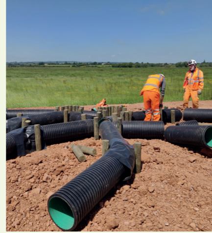
Construction of badger sett
